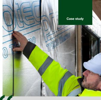
We chose to use Glidevale Protect products on this project because of their quality and reliability of performance. We work within a fabric first design and the excellent aged thermal resistance of Glidevale Protect's reflective membranes allow us to easily meet the low wall U-value requirements of both our open and closed panelled systems. "
