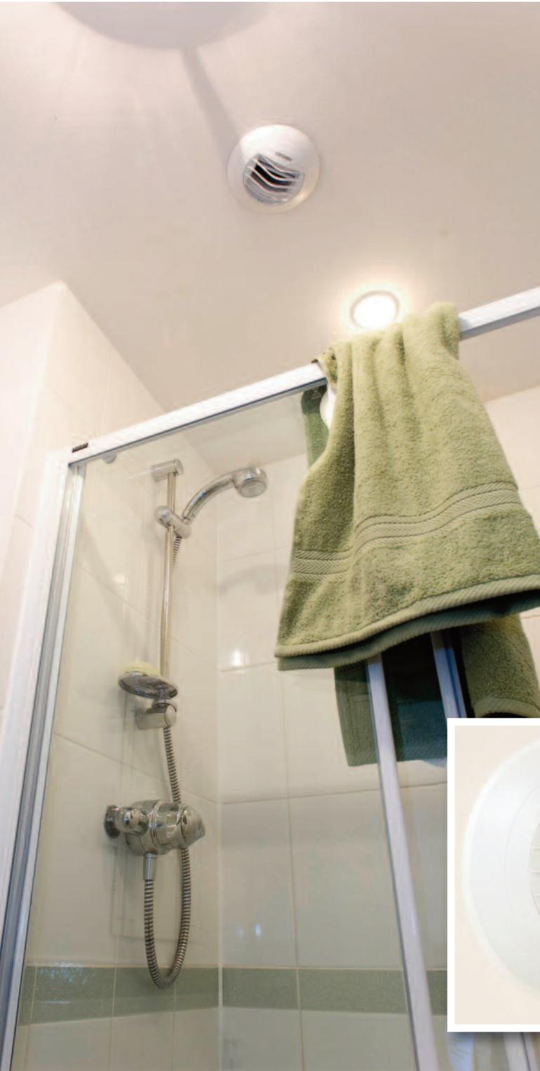
Each en-suite has a humidity sensitive extract discreetly fitted into the decorative ceiling plasterwork. The humidity sensitive extracts respond automatically to changes in relative humidity in the en-suite, and boost extraction as required to ensure a fresh, dry, draught- and odour-free environment is maintained.
