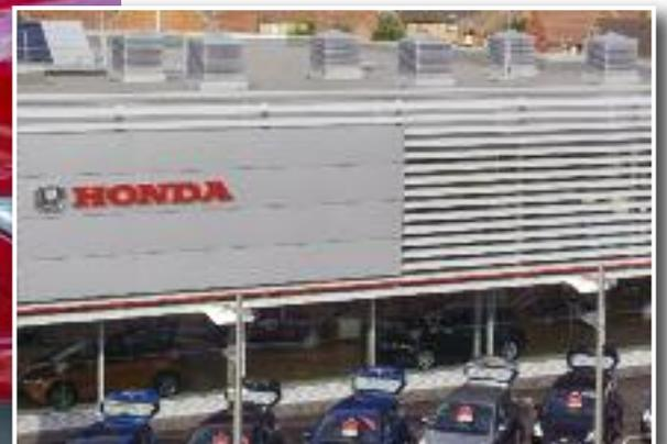
The 36 modulating wall Aircool units draw fresh air into the space on demand, maintaining internal air temperature and CO<sub>2</sub> at preset levels. Natural air movement principles, in which warm air rises, are harnessed to exhaust the warm, 'used' internal air through the six roof-mounted Airstract terminals with ceiling louvres.
